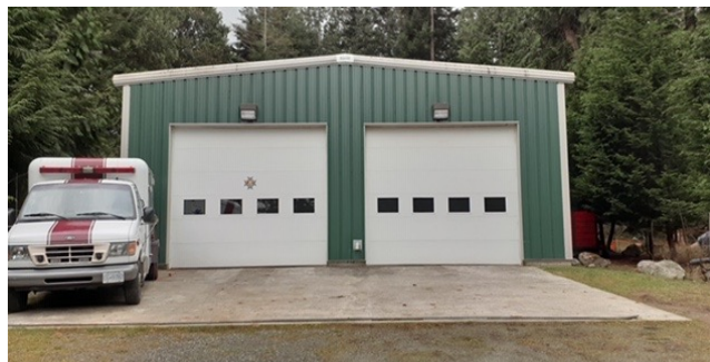
Emergency Services Building 2 (ESB#2) 646 Tumbo Channel Road (East Point)
